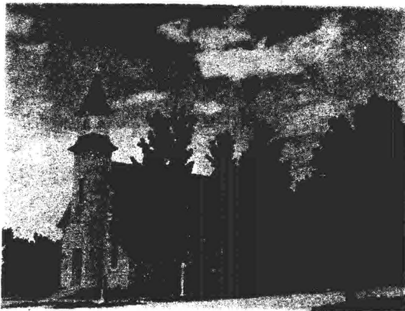
OLD SOUTH WARD CHURCH, Manti, Utah
